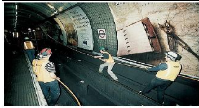
Figura B.7.– Posa in tunnel metropolitana
